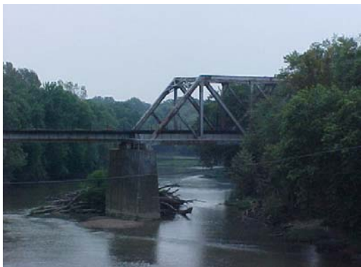
Salt River and train overpass in Shepherdsville
