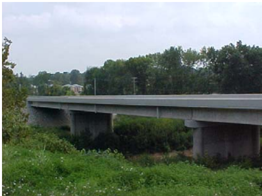
Bridge span over Floyd's Fork
