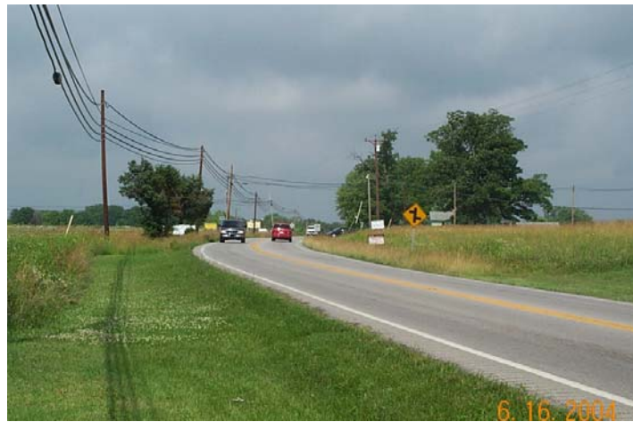
Photo No. 7 – West View at Fisher lane
