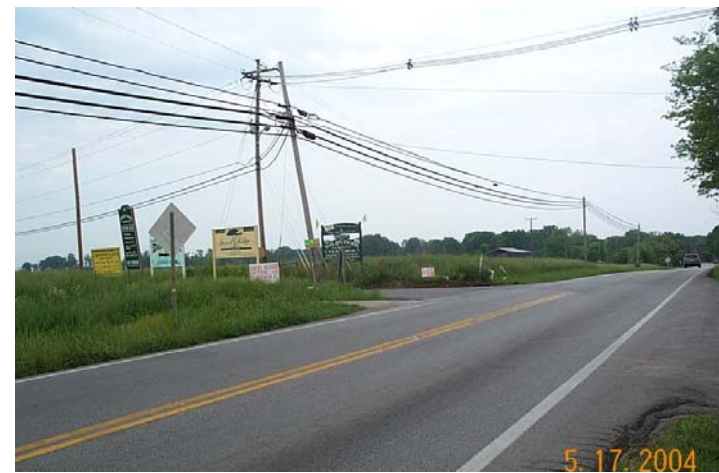
Photo No. 8 – West View at Armstrong Lane
